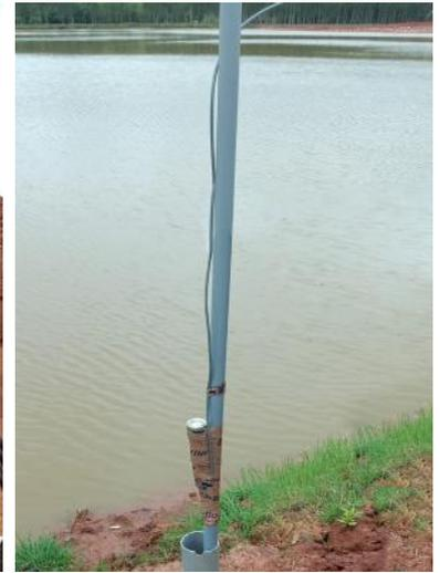
Piezometer being installed in red mud pond area
